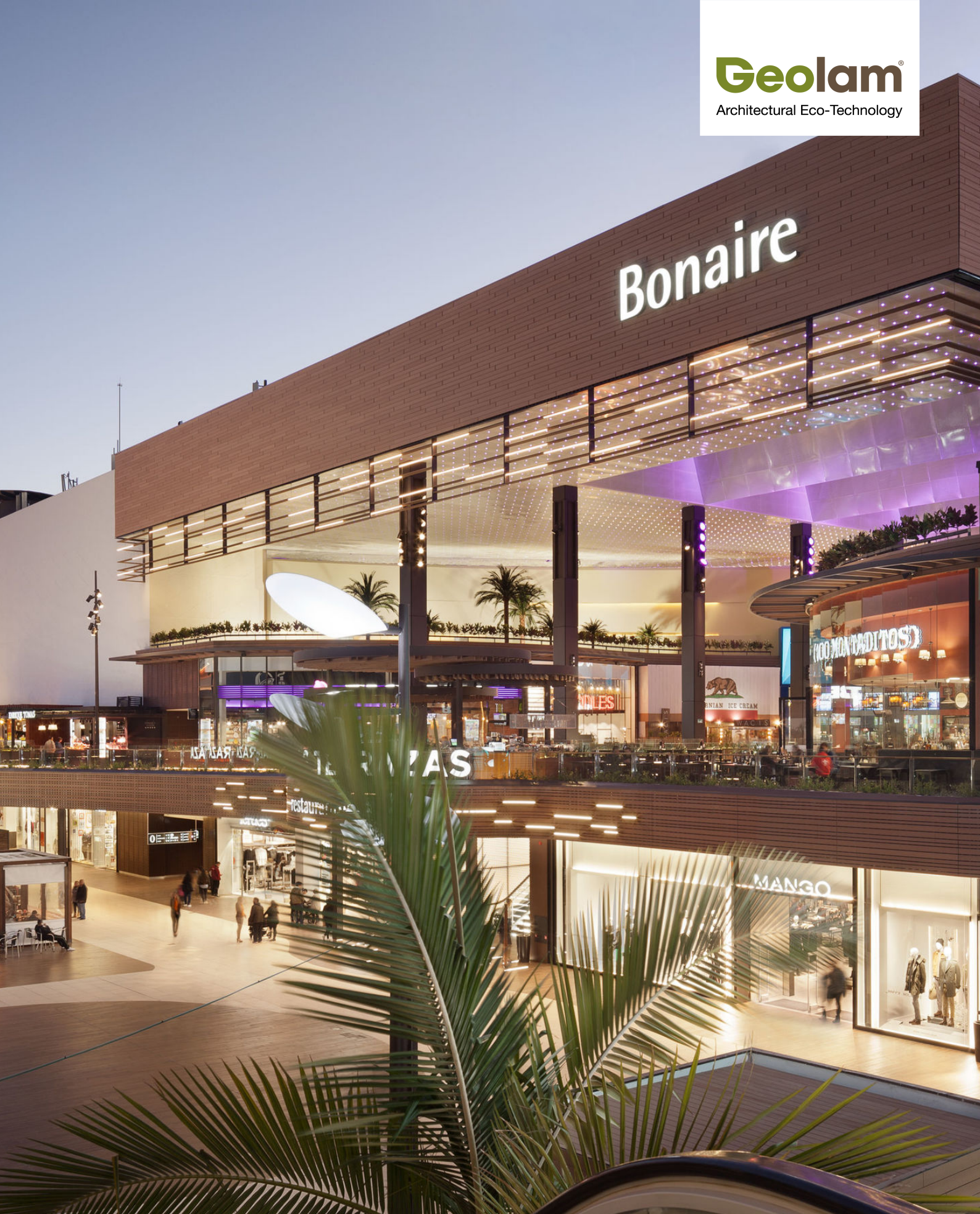
Outside Bonaire Shopping Center Building cladding
